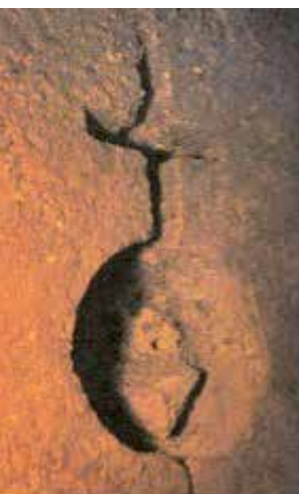
Figura 3. Troneira de orbe e cruz na torre de D. João II. / “Orb and cross” embrasure in the tower of D. João II.
